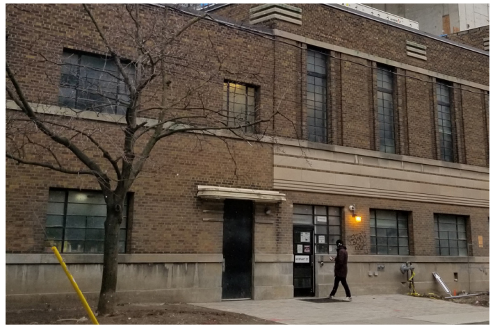
Eva's Phoenix, Toronto, in construction
