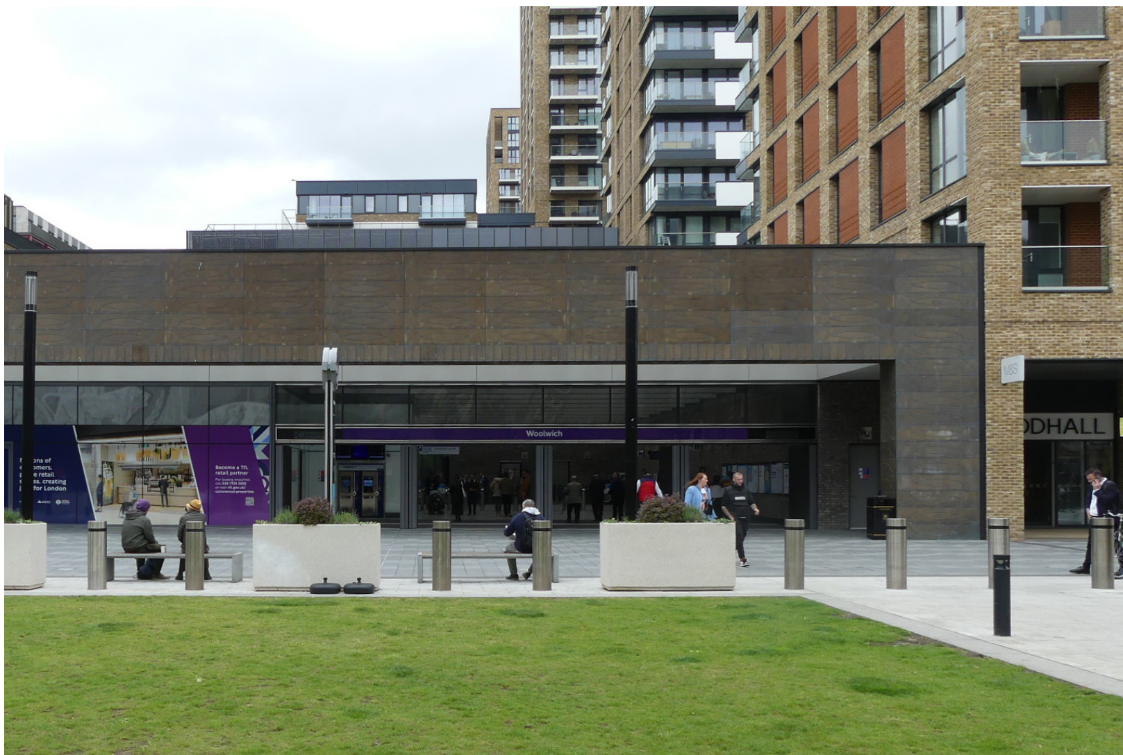
Figure 5. Station Woolwich de la Elizabeth Line
