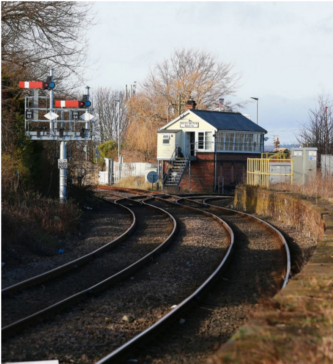
Figure 8. Northumberland rail line route, image courtesy of E-Rail
